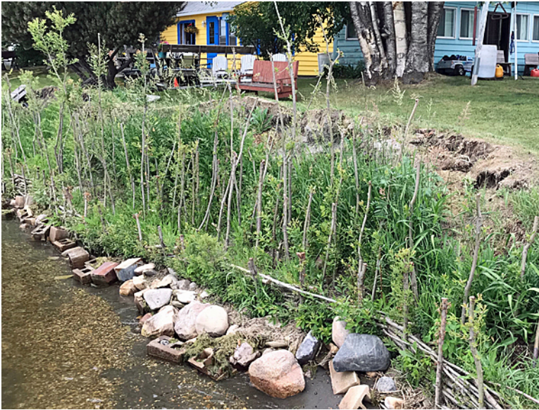
The Taylor shoreline 7 weeks after the workshop. The deeply planted willow stakes have sprouted and are rapidly growing roots, helping stabilize the shore.
