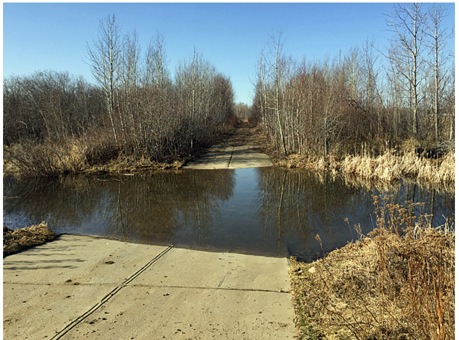
The weir at Wabamun Creek in early April 2018
