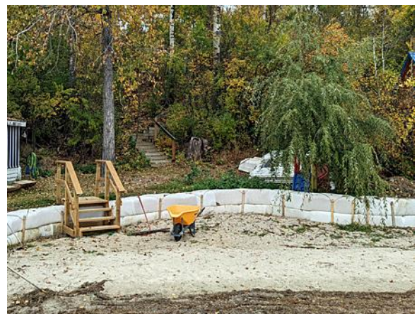
Curlex blocks installed 2022, planting in spring 2023
