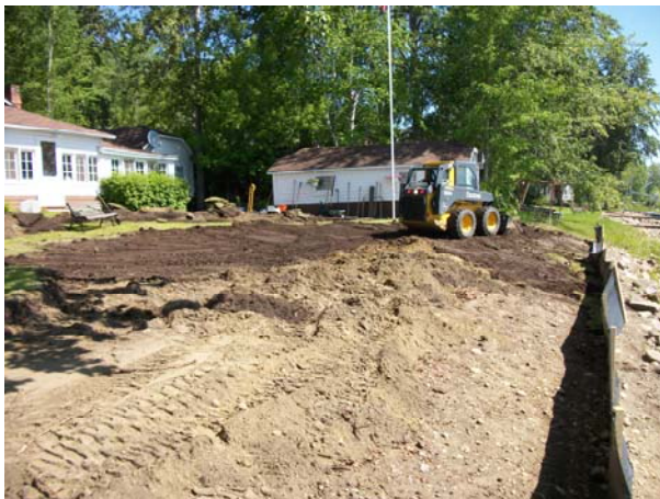
Second step: removing the top soil.
