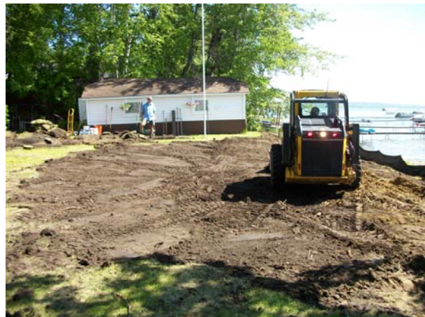
Third step: re-grading and measurement of slope to a ratio of 1:5
