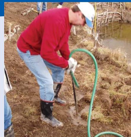
The waterjet stinger was specially designed to use high-pressure water to hydrodrill a hole in the ground to plant cuttings.
